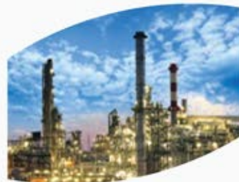
Zero Liquid Discharge (ZLD) Water Recycling
